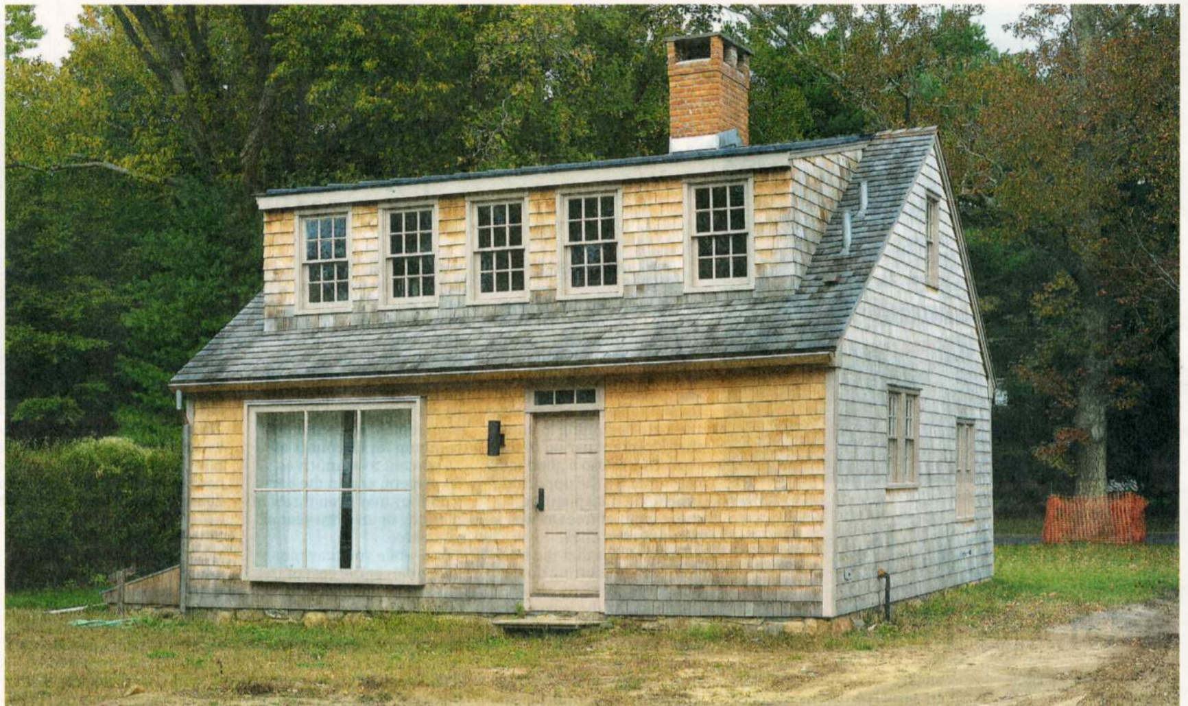
The rear view of the Hiram Sanford House.
